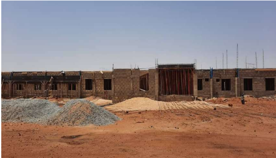
COLLEGE OF MEDICAL SCIENCE SOKOTO WORK IN PROGRESS
